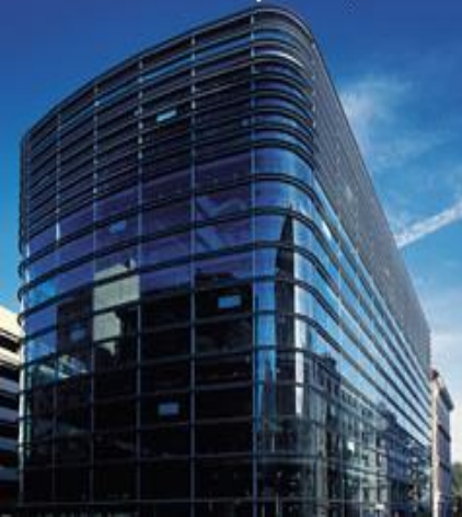
The new SGS Headquarters, Geneva
